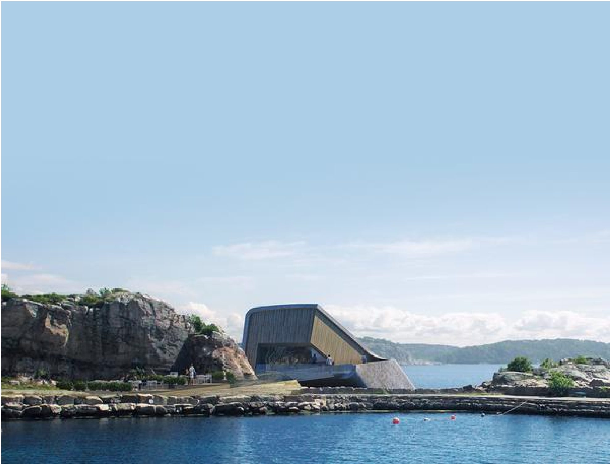
The concrete shell was cast in southern Norway. The building was constructed on a barge so that it could be lowered into the water
