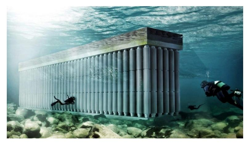
The Parthenon Seawall is a new suggestion for a floating breakwater which would protect harbours and coastlines from tidal force, turning it into electrical power.
