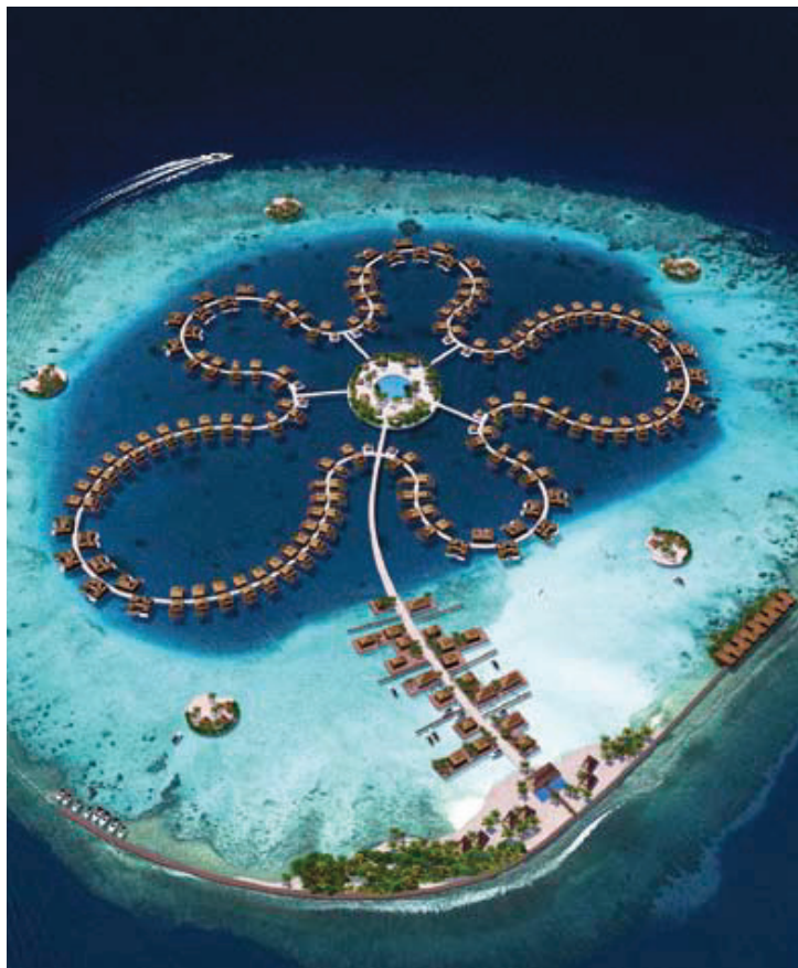
Construction of the Ocean Flower, located in the North Male atoll, is scheduled to start soon and will include villas in three different price ranges.
