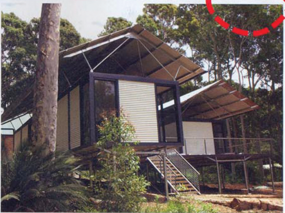
Prefabricated homes are already here. The 50m 2 e-Node comes with kitchen and bathroom. The roof, verandah and accommodation module assembled on site.
